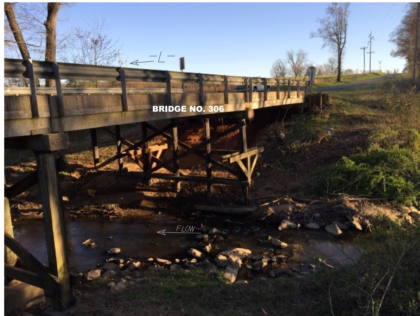
PHOTOGRAPH NO. 1: VIEW LOOKING SOUTH FROM END BENT NO. 2.
